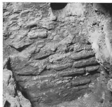
Fig. 106 — S. Lorenzo f.l.m. Basilica maior , dig 7, facade wall, east face, top part (Photo: Sansaini).
